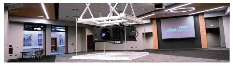
In addition to brilliant image quality, the NP-PX2000UL provides quiet and unobtrusive integration. To capitalize on this, SVT worked with Draper to create an enclosure that can raise and lower the projector from a panel in the ceiling, providing a solution that melts into the environment when not in use.
